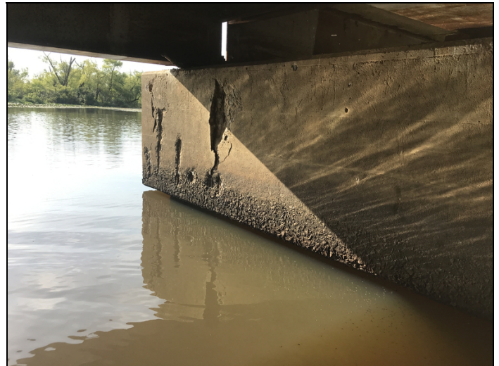
Bent 3 cap spalls with exposed rebar
