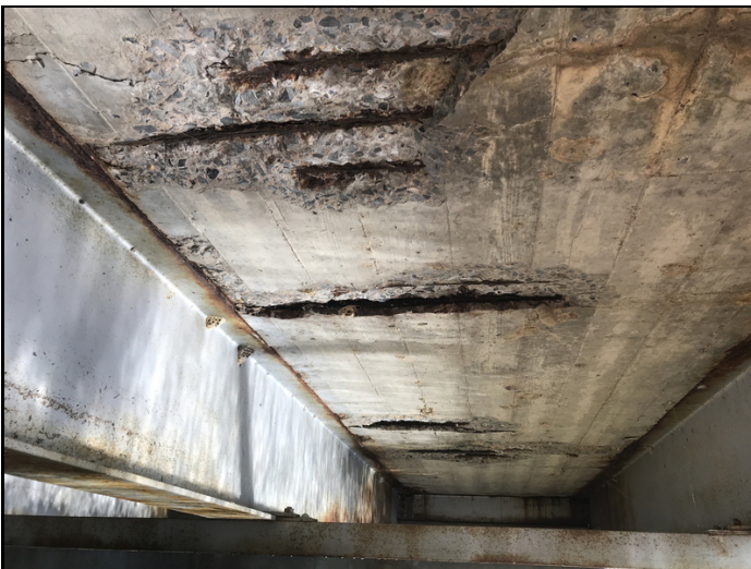
Span 2 soffit between beams 1&2, large spalls with section loss to exposed reinforcing steel.
