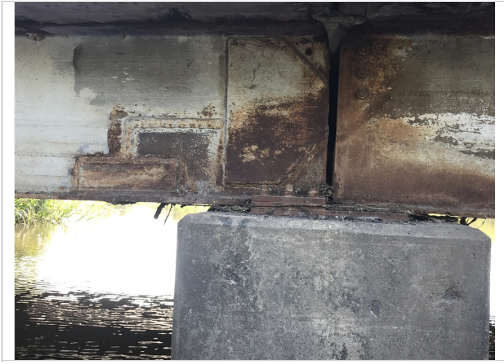
T-splice repair span 2 beam 5
