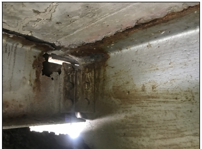
Span 1, bent 2, beam 2: upper web with deep pitting and diaphragm with large hole due to corrosion action.
