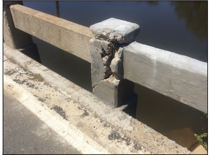
Span1 right bridge rail damaged.
