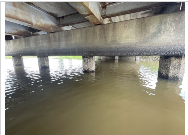
Heavy abrasion to piles at bents 2 and 3
