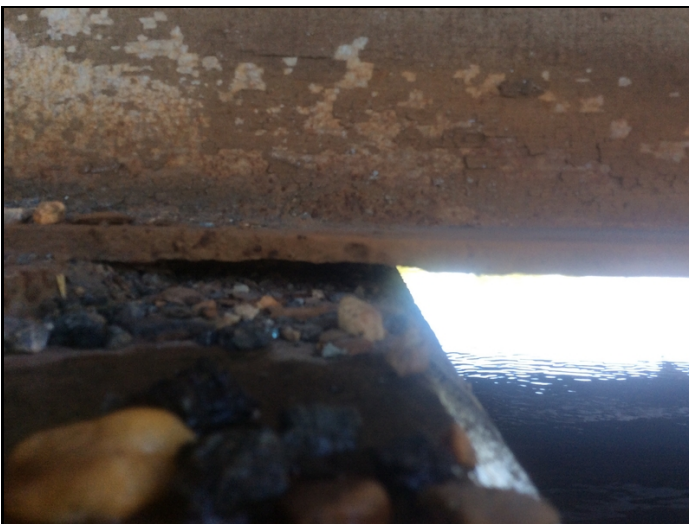
Bent 3 span 3 beam 5 1/4" pitting to lower flange.
