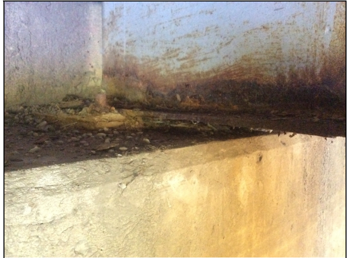
Bent 1 span 1 beam 2. 3/16" pitting to bottom flange.
