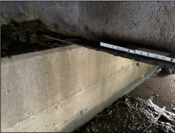
Span 1 bent 1 beam 3, 1/4" section loss to bottom flange
