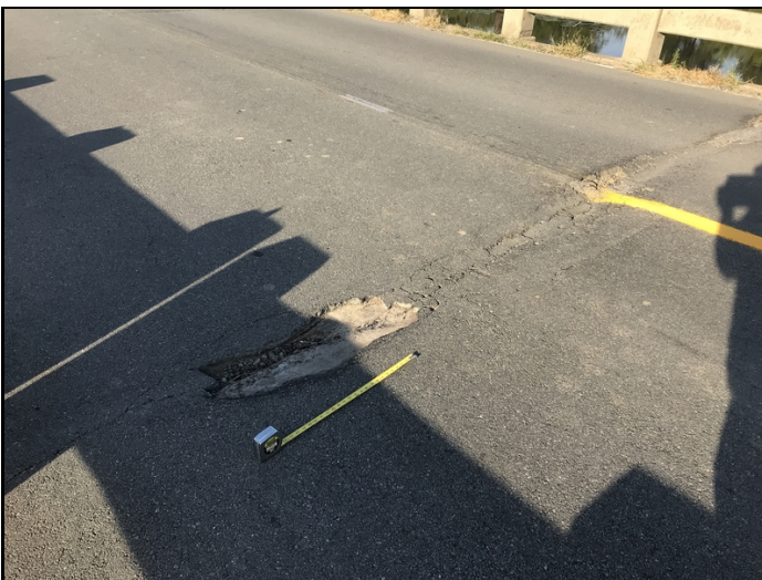
Spalls in asphalt overlay at bent 2
