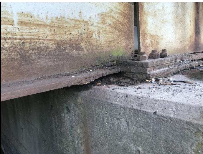
Span 1, bent 2, beam 5: Bottom flange with measurable section loss near bearing.
