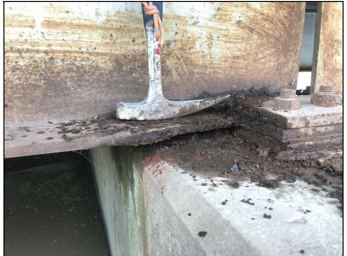
Span 1 at bent 2, beam 5: bottom flange has lost half it's section due to corrosion at the bearing area
