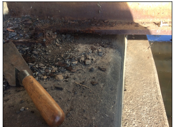
Bent 4 span 3 beam 1, 3/16" pitting to bottom flange.
