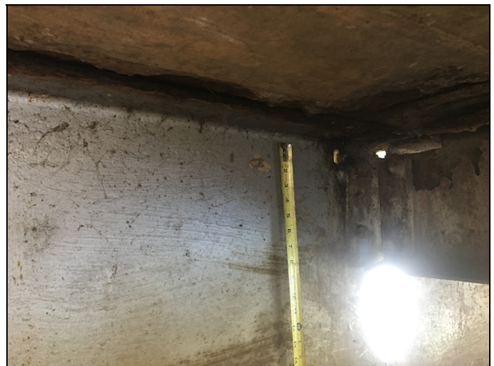
Bent 2 span 1 beam 2 hole in the upper web.
