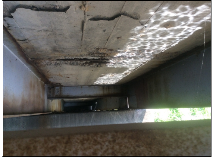
Span 2 soffit spalls with exposed rebar. Common all spans.
