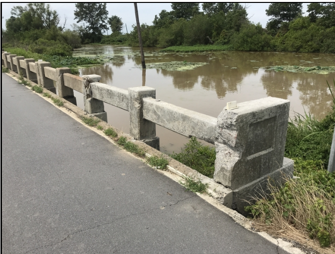
Right rail: the first 3 posts have been damaged due to traffic impact
