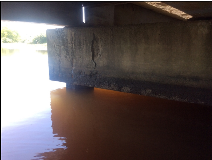
Bent 3 cap back left side spalls with rebar.
