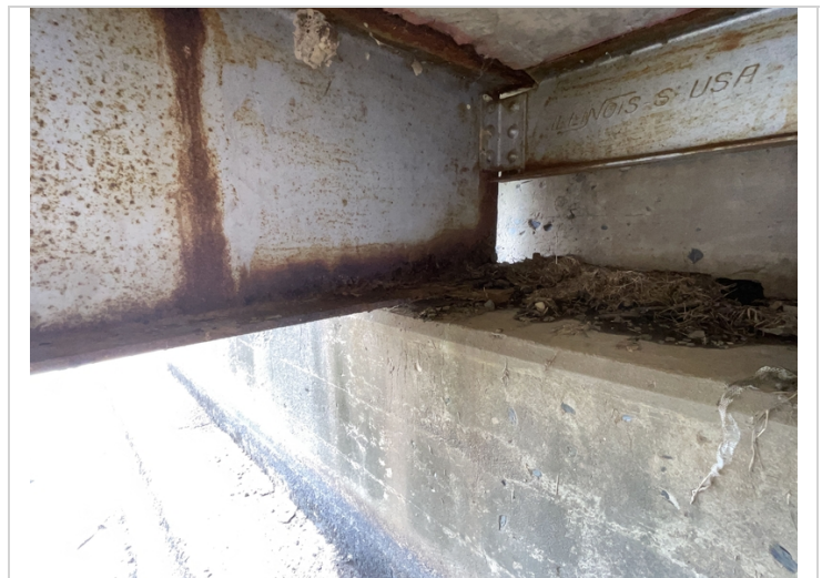
Bent 4 beam 1 lower flange and bottom of the web has pitting up to 3/16"
