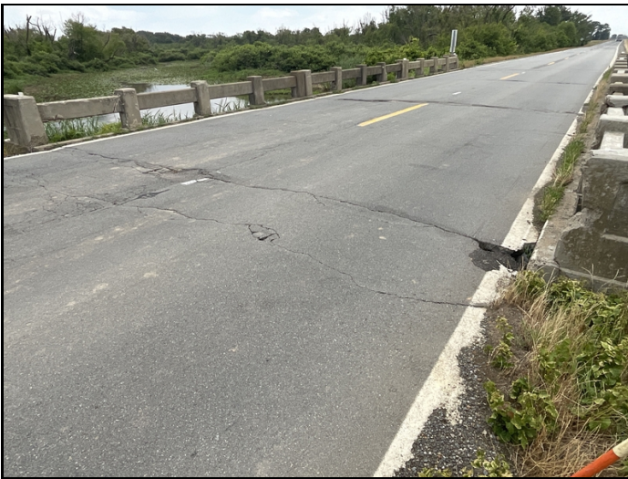
Potholes at joints
