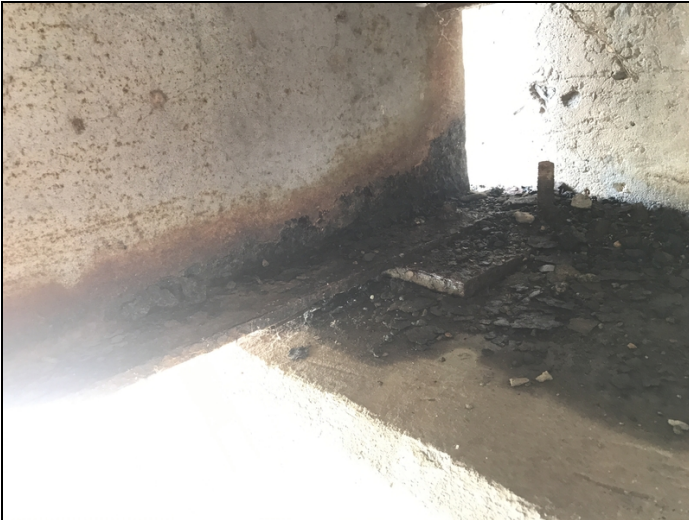
Span 4, girder 1: Section loss to the lower web and bottom flange.
