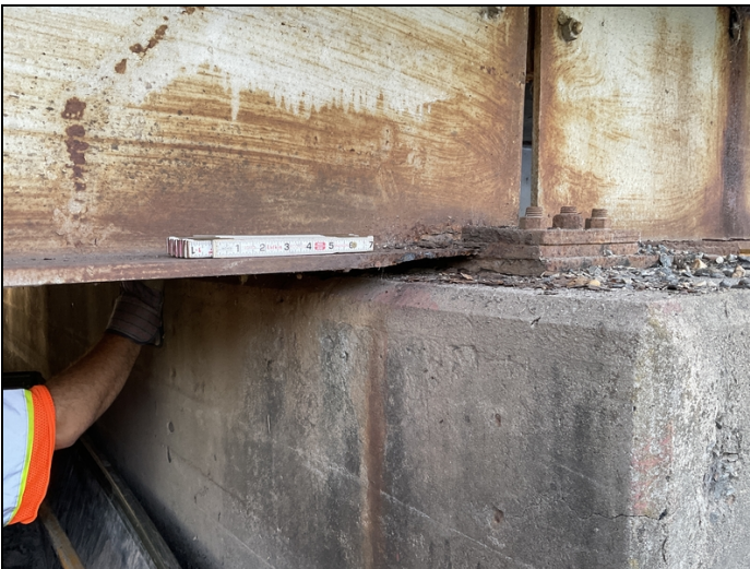
Bent 2 span 1 beam 5, 1/4" section loss to bottom flange at bearing area.
