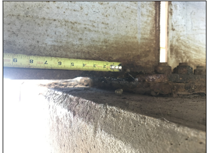
Span 2 beam 2 at bent 3, 3/16" section loss to bottom flange
