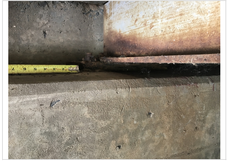
bearing at Beam 4 at bent 4 laminating rust
