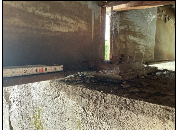
Bent 3 span 2 beam 1 bottom flange on right side is down to knives edge. Worse case.
