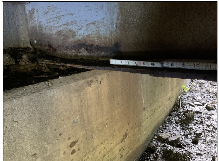
Bent 1 beam 2 1/4" section loss to bottom flange. 1/8 in lower web
