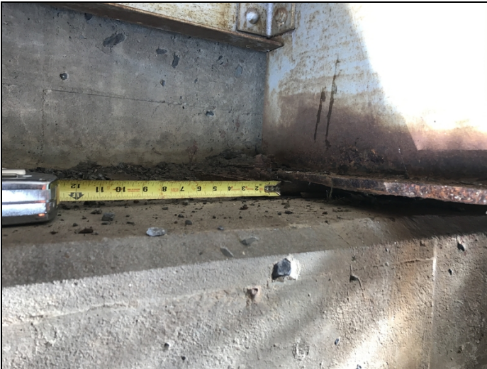
Beam 2 Span 3 at bent 4. 3/16" section loss to bottom flange
