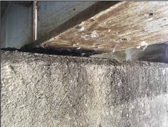
Span 3 girder 1: common condition to majority of beams with section loss to the bottom of the lower flange
