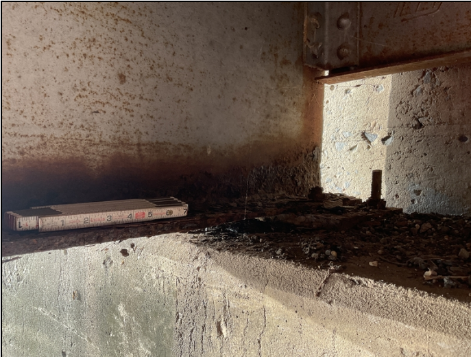
Bent 4 span 3 beam 1, 1/4" section loss to bottom flange.
