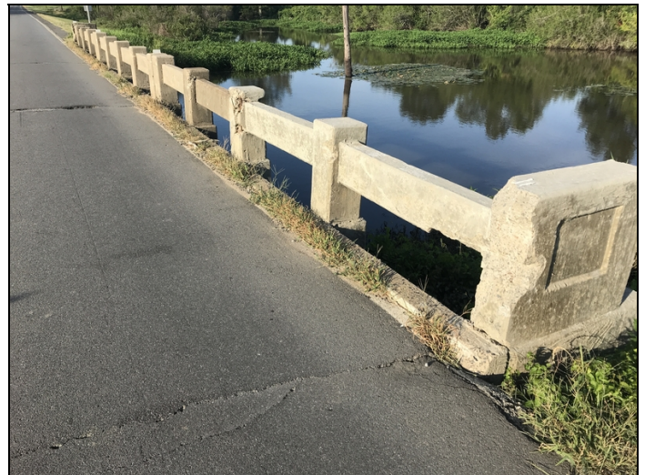
Span 1 right bridge rail has traffic damage
