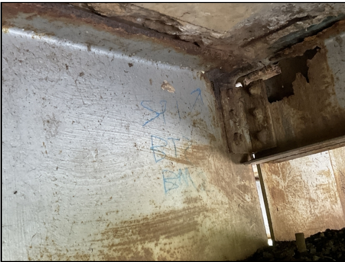
Bent 2 sp1 bm 2 hole in upper web
