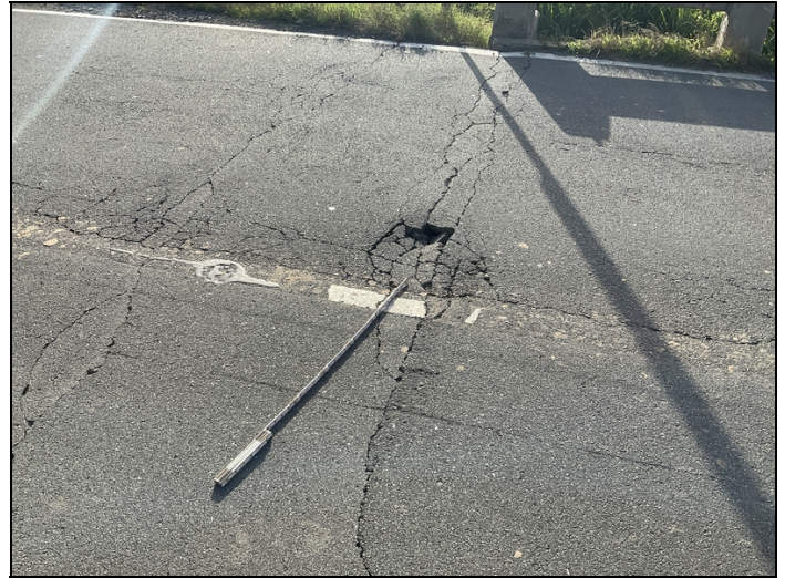
Void under approach roadway at bent 1. Asphalt is cracked and settling.
