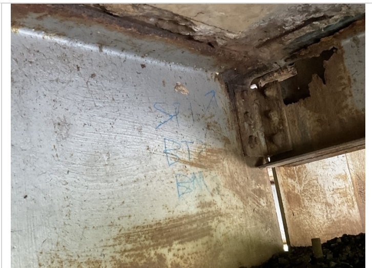
Bent 2 sp1 bm 2 hole in upper web
